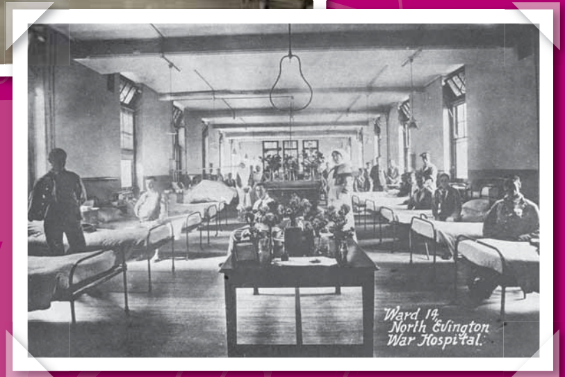
1914 – Nightingale ward The ward layout was designed by Florence Nightingale around 1860. They were 87 feet long by 24 feet wide with two central coal-fired stoves and electric light.
